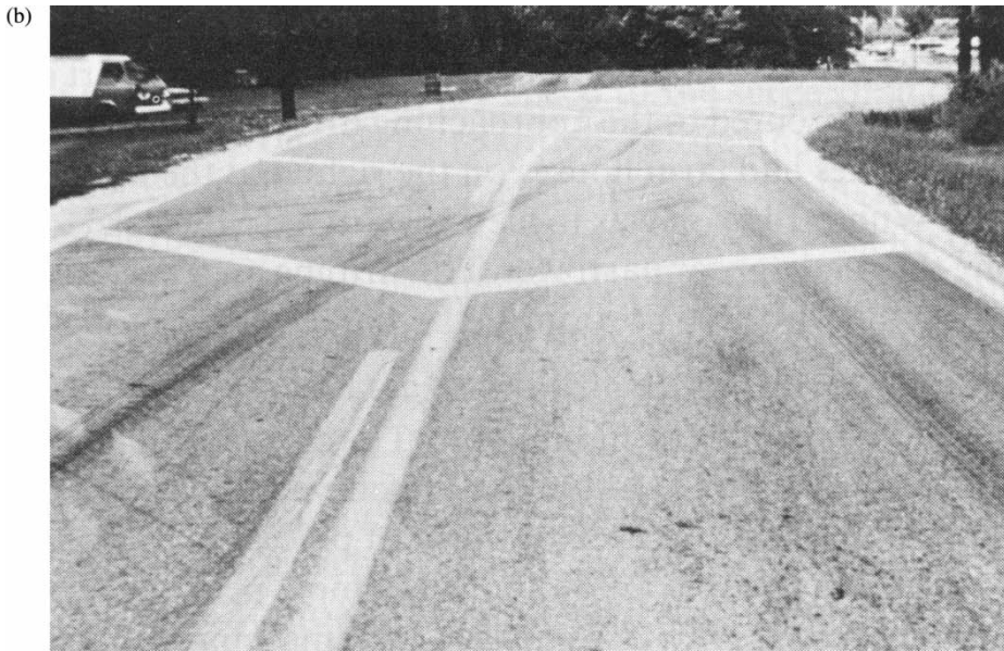
Figure 2. Techniques for slowing drivers at dangerous curves from Shinar et al. 1980, pp. 268–269: a) increasing visual angle of the inside curve; b) using the Wundt illusion to make the road seem narrower; c) decreasing the distance between adjacent transverse stripes on the road; d) posting a warning sign. Figure reprinted with permission of Taylor & Francis Ltd. ( http://www.tandf.co.uk ).
